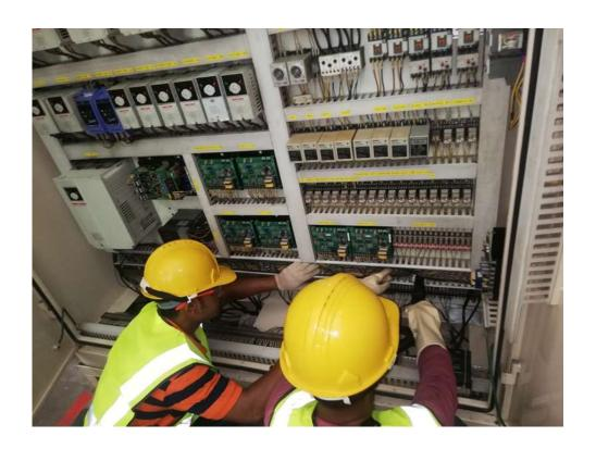
The physical connections between Clocks, IEDs, Switchgear, Circuit Breakers and Bay Controllers are often located in **small**, **hard-to-reach** panels, **making it difficult to connect** other devices
